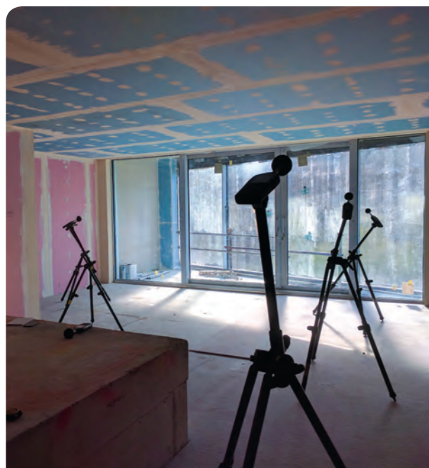
Measuring how much noise passes through a building façade using a large scale mock-up
