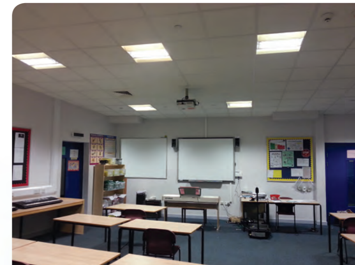
BRE evaluated lighting conditions in areas of a school lit by two types of ceiling recessed fluorescent luminaires
