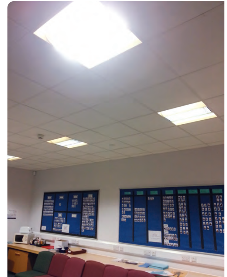
Bright light sources can cause disability glare, which can be avoided by correctly aiming or shielding the lamps
