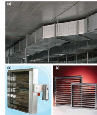
Figure 1: (a) Fire-resisting duct system, (b) steel fire damper, (c) intumescent fire damper
